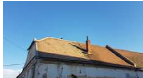
Roof and exterior repairs—Arapamesu Day Center
