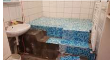
Bathroom project, creating a shower space
